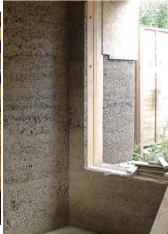
Cast-in-situ hempcrete forms a continuous mass, reducing thermal bridging.
