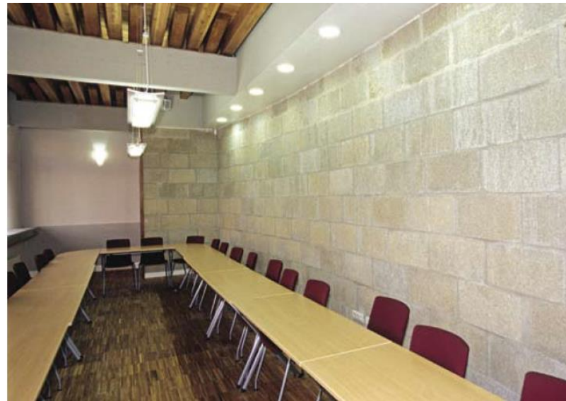
Hemp lime construction, Rachel Beaven, 2008
