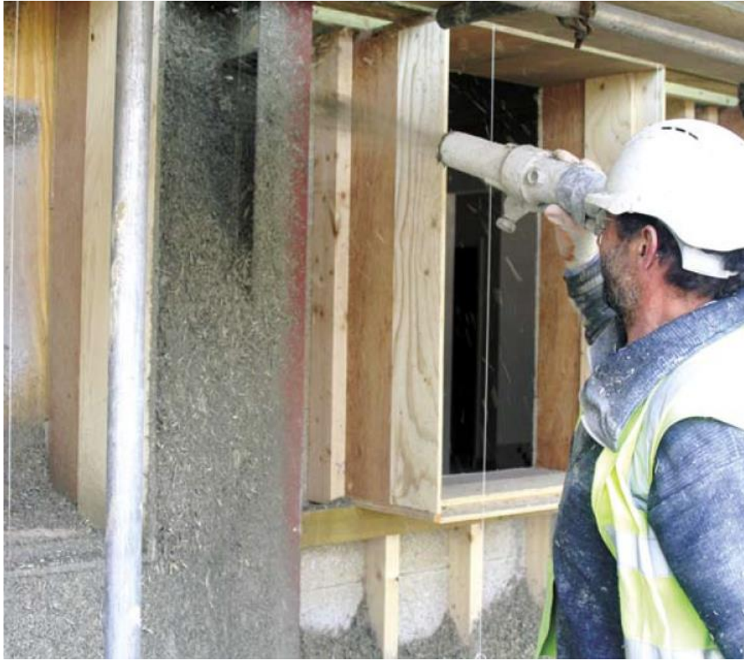
Hemp lime construction, Rachel Beaven, 2008
