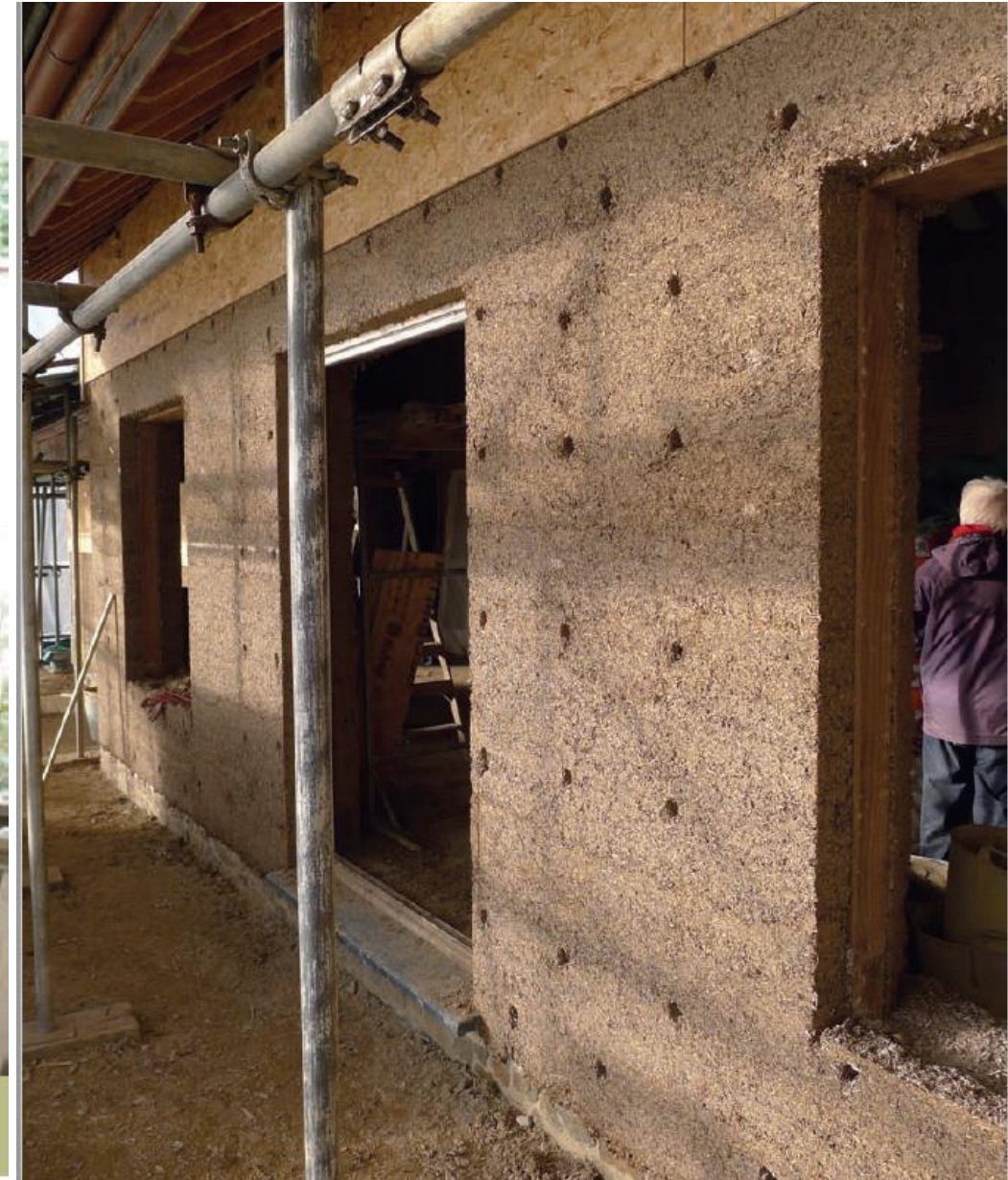
Cast-in-situ hempcrete forms a continuous mass, reducing thermal bridging.
